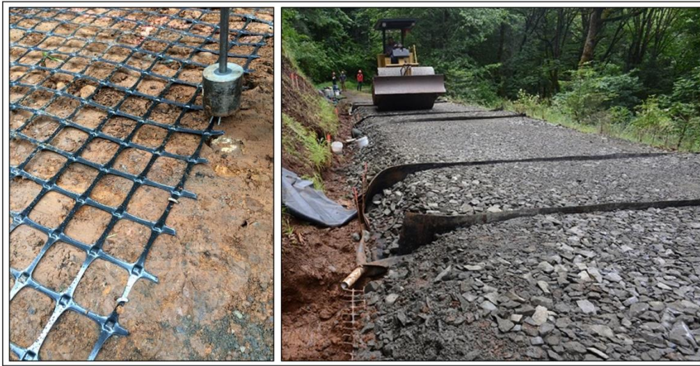
Figure 1. Test track construction: geogrid placement over subgrade (left); buried runoff collection flumes in roadway (right)
